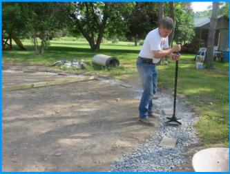
Tamp the crushed stone between pavers.
